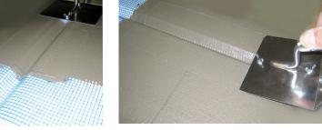
After coating your groove with base coat, place a workable width of mesh on top of the precut groove. Then move the matching groove sled forward to imbed the mesh and remove any excess base coat. The sled will push the mesh into your base coat evenly, filling the precut groove and eliminating any snags or cuts in the mesh that might occur
